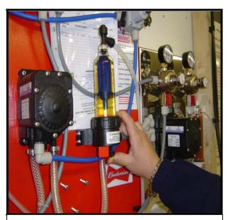
3) If a Fob detector is fitted to the line, put it into 'clean mode' by pushing the knob upwards and then hold it in place with the Red over ride switch
